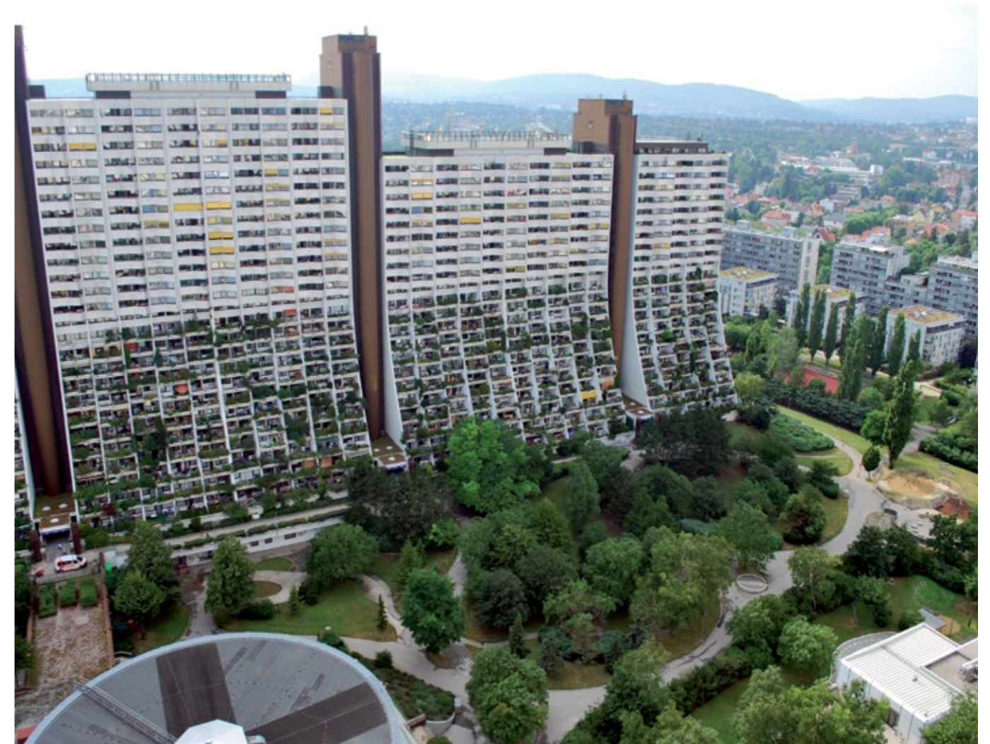
Alt-Erlaa housing estate from 1970ties | cg
